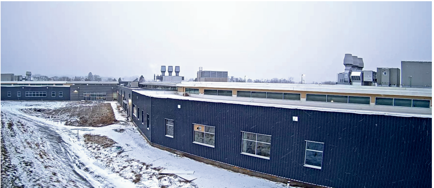
South Side of Building, Facing North
